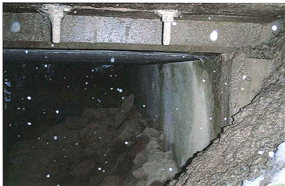
CK 2128 Abutment Right Bank
