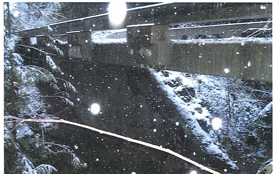
CK 2128 Crossing Upstream
