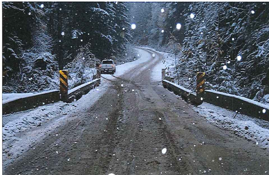
CK2128 Approach Left Bank
